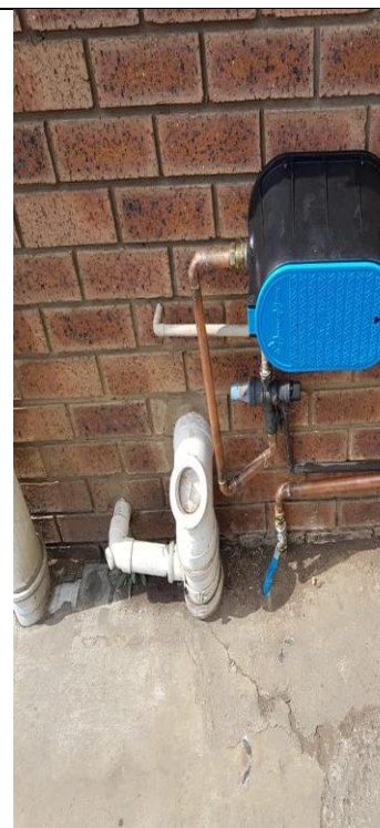
Installing Water Meters
