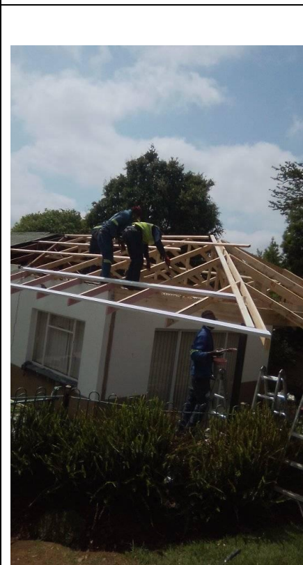
Roofing a House
